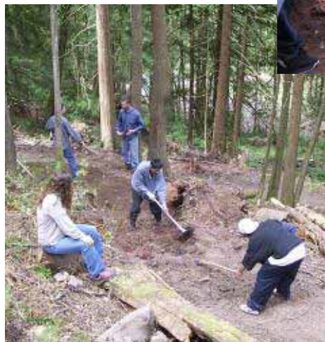
Parrott Creek Ranch trail crew realigned and surfaced a section of Hopkins Trail to make it an easier walk for more visitors to the forest.
